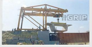
Gantry / Goliath Cranes are adapted to applications where overhead runways would be very long, costly to erect, and difficult to maintain in alignment. Where the installation is only temporary, a gantry crane can be moved to a new location with less trouble or expenses than
