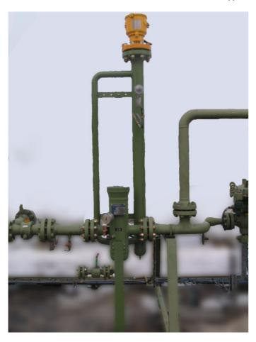
They combine the filter function and heater and are most often installed upstream of an expansion valve.
